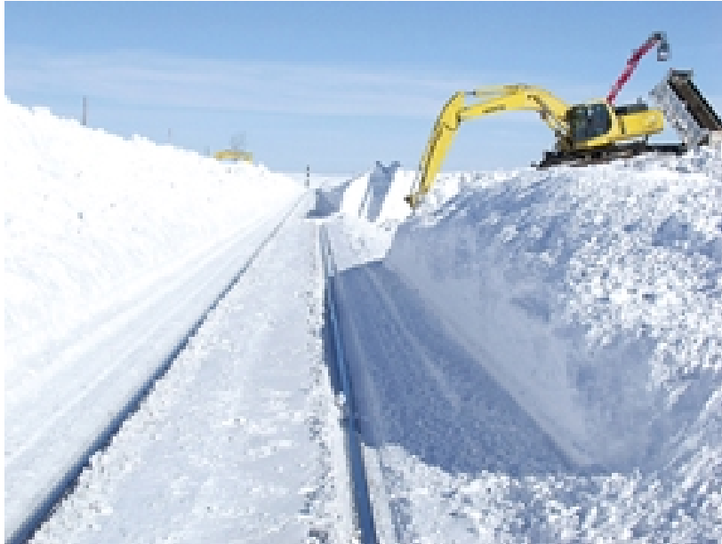
Railroad snow removal between Minot and Williston. Amtrak train had to stop near Epping North Dakota backing up to Williston North Dakota, 15 miles to the southwest. Photo taken by Tim Pederson, Williston Daily Herald.
