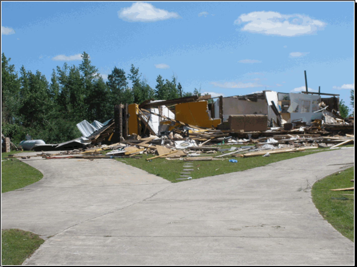
Home destroyed by EF-3 tornado along County Road 32 in northern Choctaw County Alabama on April 27, 2011. Photo by NWS Forecast Office Mobile / Pensacola.
