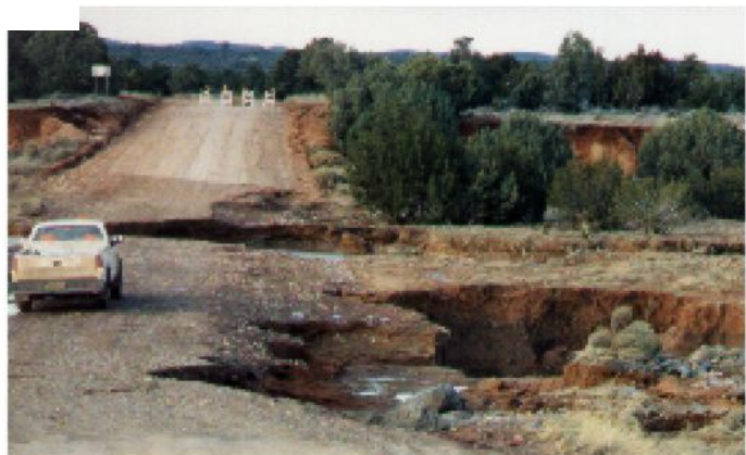
Floodwaters often conceal damage to the roadbed.
