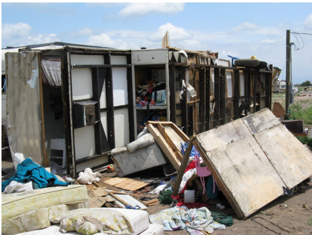
Flipped/Destroyed trailer home, Alton, TX, May 16, 2008
