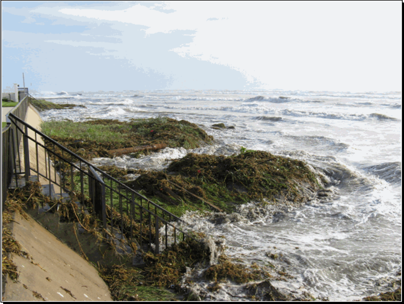
Waves reaching the seawall at the Travelodge Hotel on Gulf Boulevard, South Padre Island, TX, 845 AM September 12th, 2008
