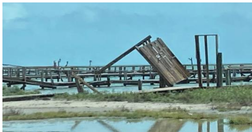
Left: Pier and wood frame damage (wind) in Port Mansfield. Right: Industrial building damage in Raymondville.
