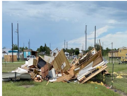
Extensive damage to colonias east of Edinburg, TX, following Hurricane Hanna in July, 2020.
