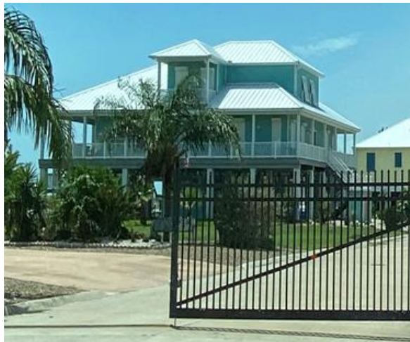
Above: This well built home in Port Mansfield (Willacy County, TX) survived 90 mph winds with Hurricane Hanna in 2020.
