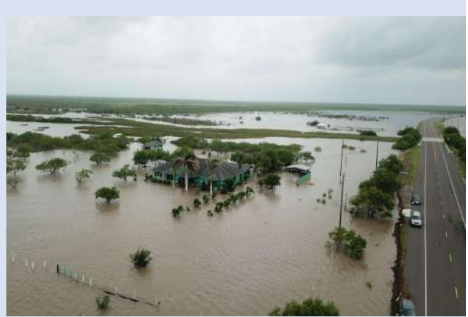
The Los Fresnos Overflight (drone) photo. Provided by Cameron Co. Office of Emergency Management.
