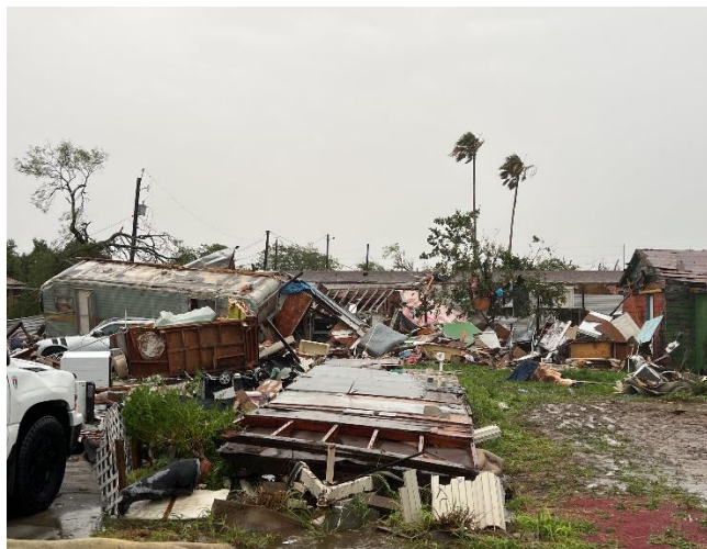
Left: Complete roof decking damage to the El Castile Condominium roof decking on South Padre Island, early on May 9 th , 2023. Right: Demolished very substandard/unanchored structures in Laguna Heights from an EF1 tornado early on May 13 th , 2023.
