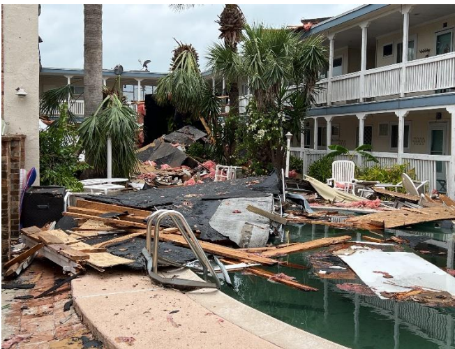
Left: Complete roof decking damage to the El Castile Condominium roof decking on South Padre Island, early on May 9 th , 2023. Right: Demolished very substandard/unanchored structures in Laguna Heights from an EF1 tornado early on May 13 th , 2023.
