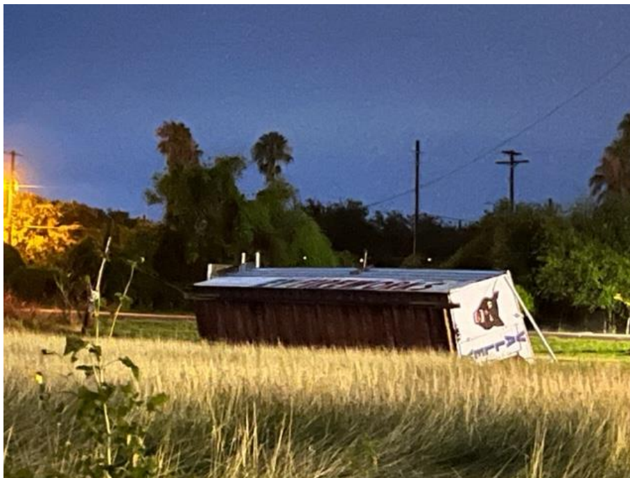
Above: Flipped fireworks stand in east San Benito, June 4, 2023, from wind gusts estimated at 60 mph. The stand was facing directly into the north wind and not securely anchored.
