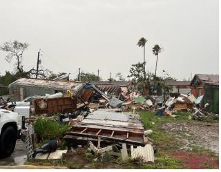
*Left*: Complete roof decking damage to the El Castile Condominium roof decking on South Padre Island, early on May 9<sup>th</sup>, 2023. *Right*: Demolished very substandard/unanchored structures in Laguna Heights from an EF1 tornado early on May 13<sup>th</sup>, 2023.
