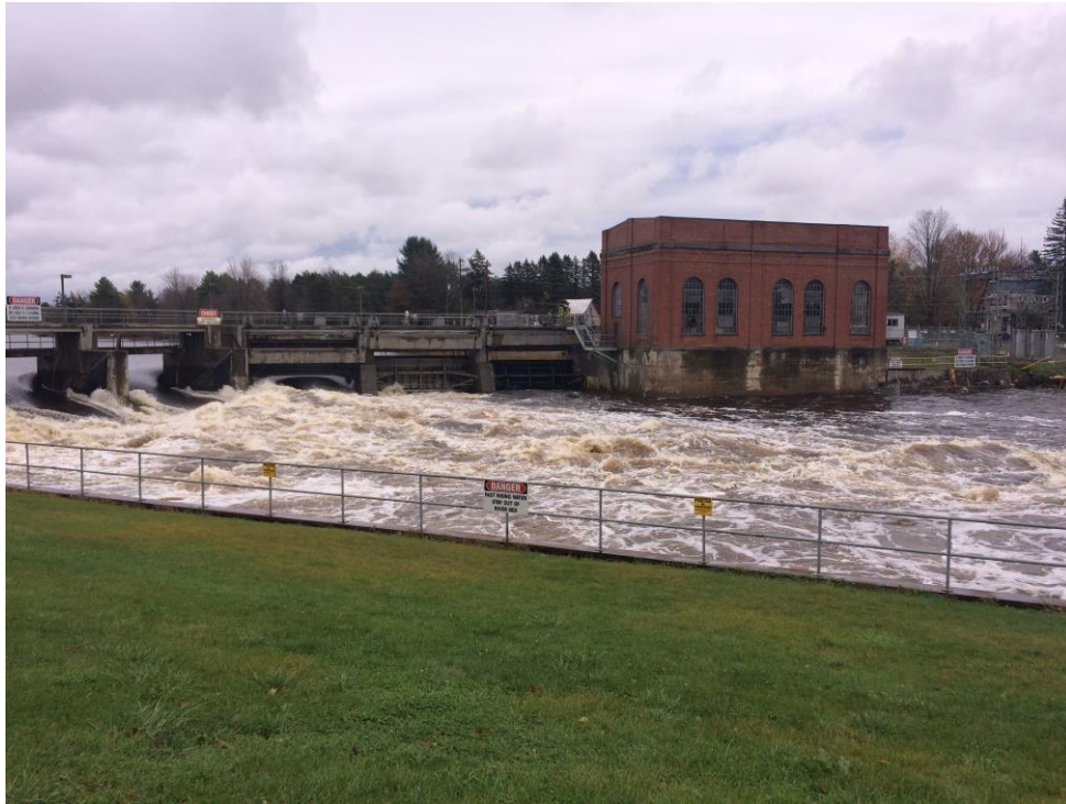
Figure 4: Hydro Dam on the Oswegatchie River in Heuvelton, NY on 3 November, 2017.
