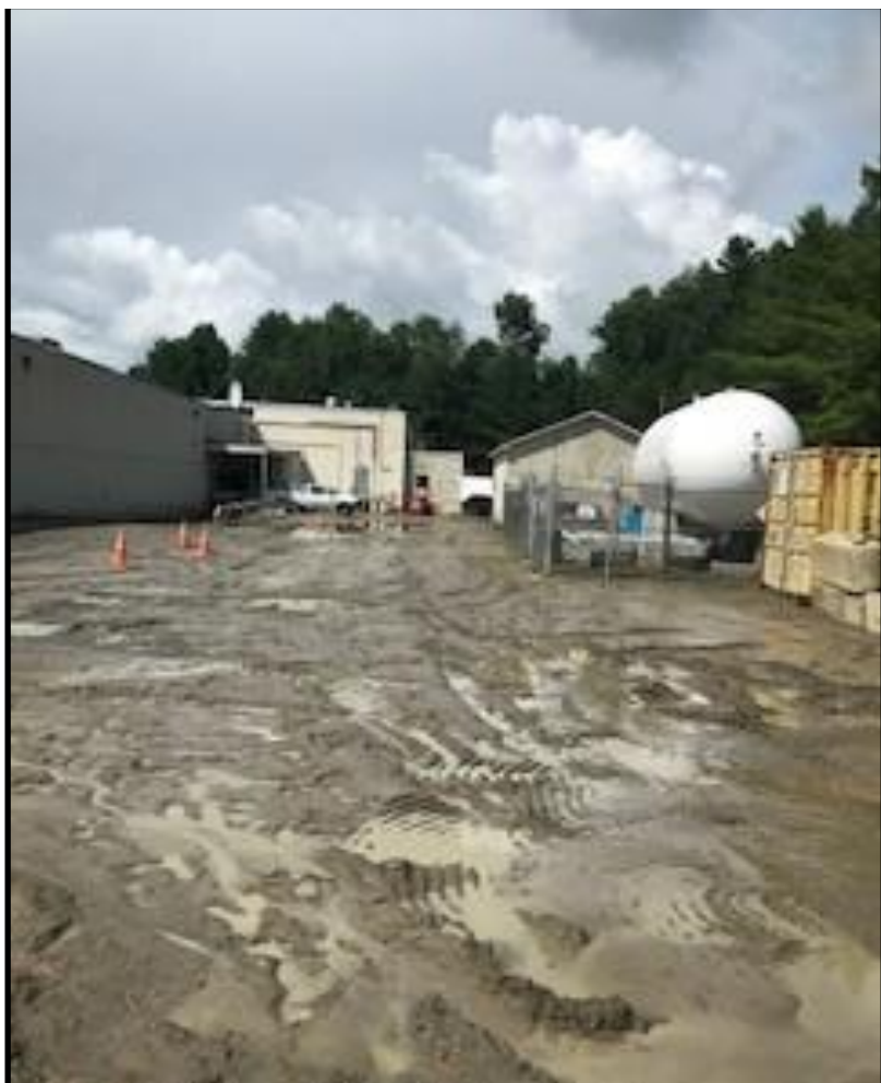
Figure 4. Mud slide that occurred in St. Johnsbury, VT after heavy rains on the morning of July 14. Photo courtesy of State of Vermont, Division of Fire Safety.
