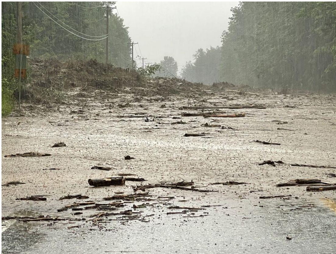
Figure 5: A close-up view of a landslide blocking U.S. Route 4 in Killington, VT during the early evening of July 7, 2023. Up to 5 inches of rain fell in this area leading to areas of significant to severe flash flooding. Photo courtesy public.
