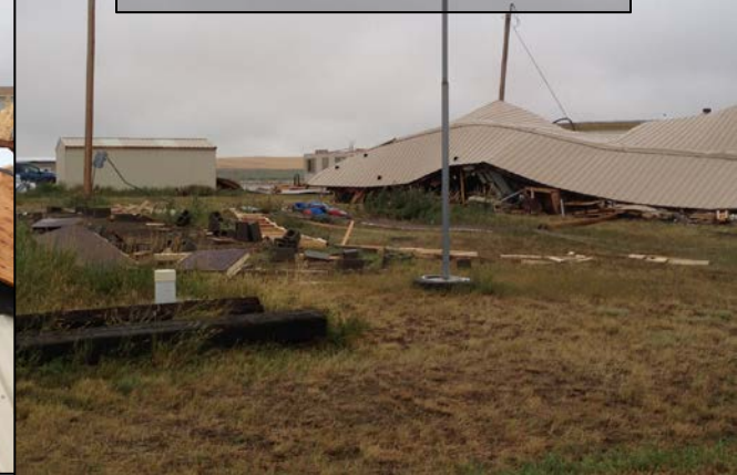
Mobile Home Destroyed
