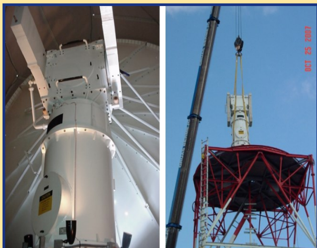
Doppler Radar Pedestal Replacement
