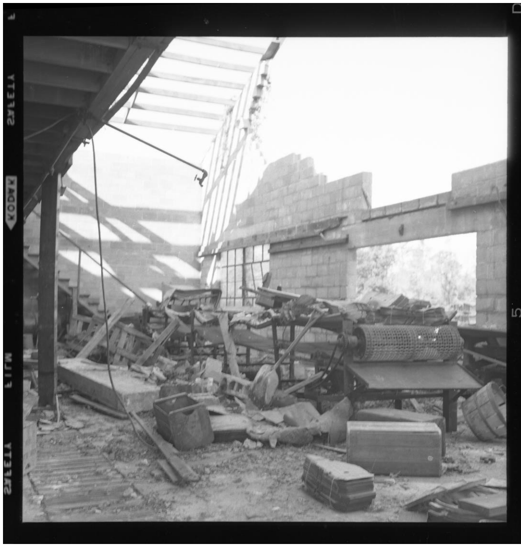
Damage to the GW Trask packing shed from Hurricane Gracie. Image courtesy of Beaufort County Library, SC.
