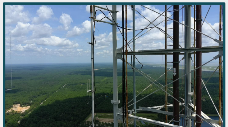
Below Image: Damaged Antenna
