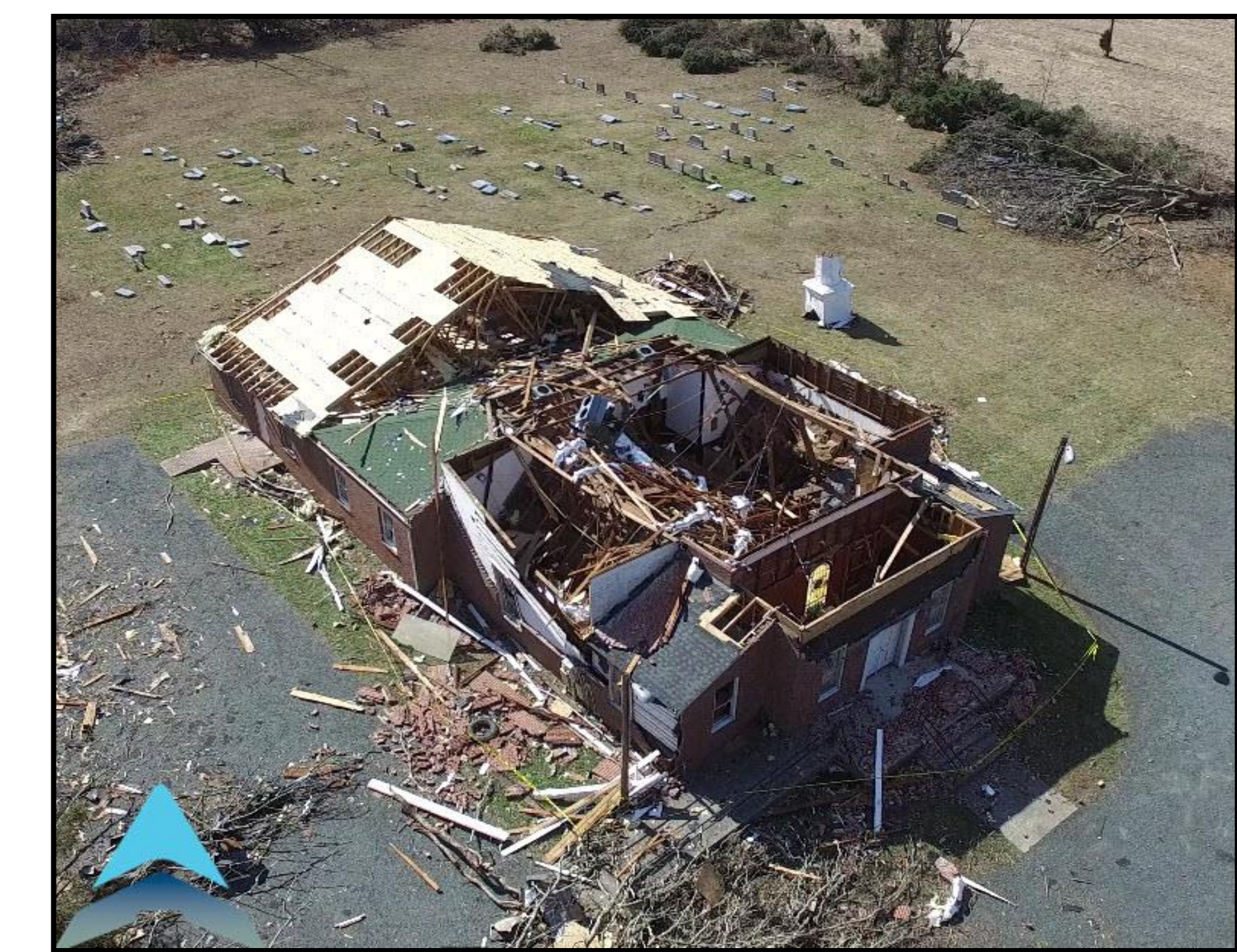
Figure 5: Aerial image of EF2 damage to Central Church near Appomattox, VA. Courtesy Autonomous Flight Technologies
