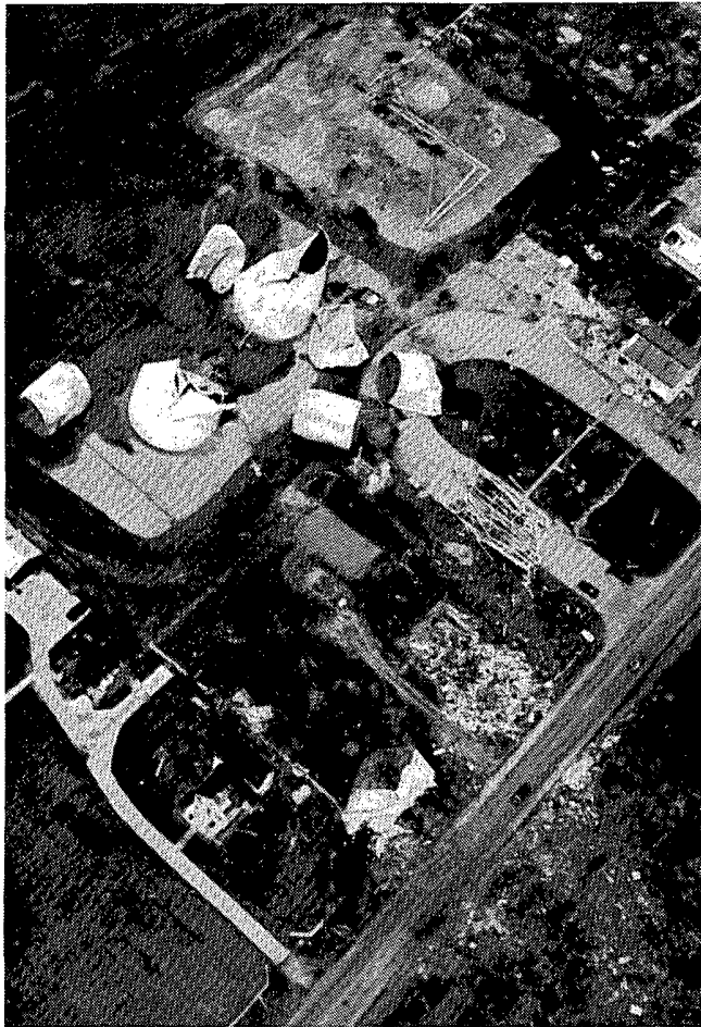
Destruction caused by the Wheatland Tornado included this petroleum tank farm (left and above) on the west edge of Niles, Ohio. Some of the tanks were bounced a considerable distance.
