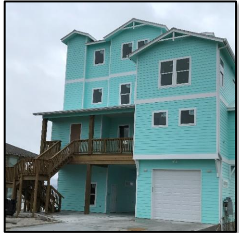
Above: This well built home in the community of Copano Village in Aransas County, TX survived Hurricane Harvey in 2017.
