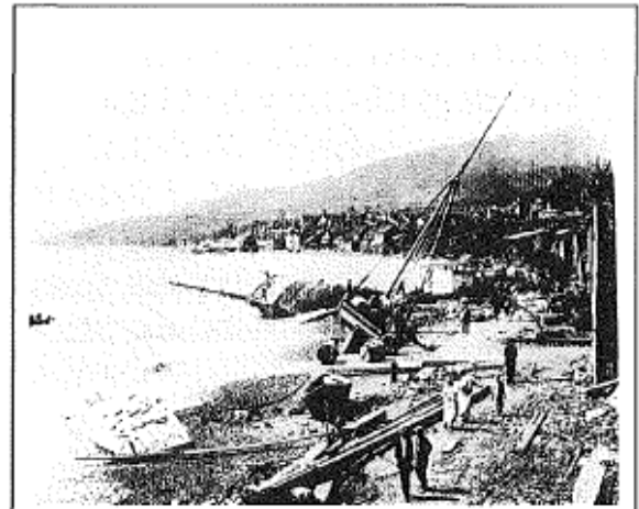
Damage caused by a 3–4 metre tsunami wave at Saint-Pierre, 5 May 1902.
