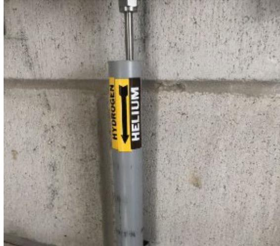
*Figure K-9: Acceptable Markings for Helium/Hydrogen Tubing*
