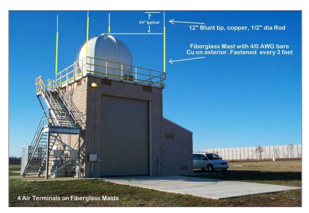
Figure 2-3. Lightning Protection for Upper Air Buildings (Franklin Rod Design)
