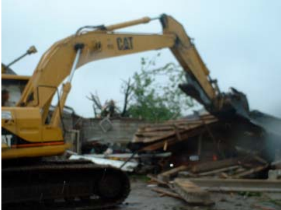
Looking north to destroyed garage
