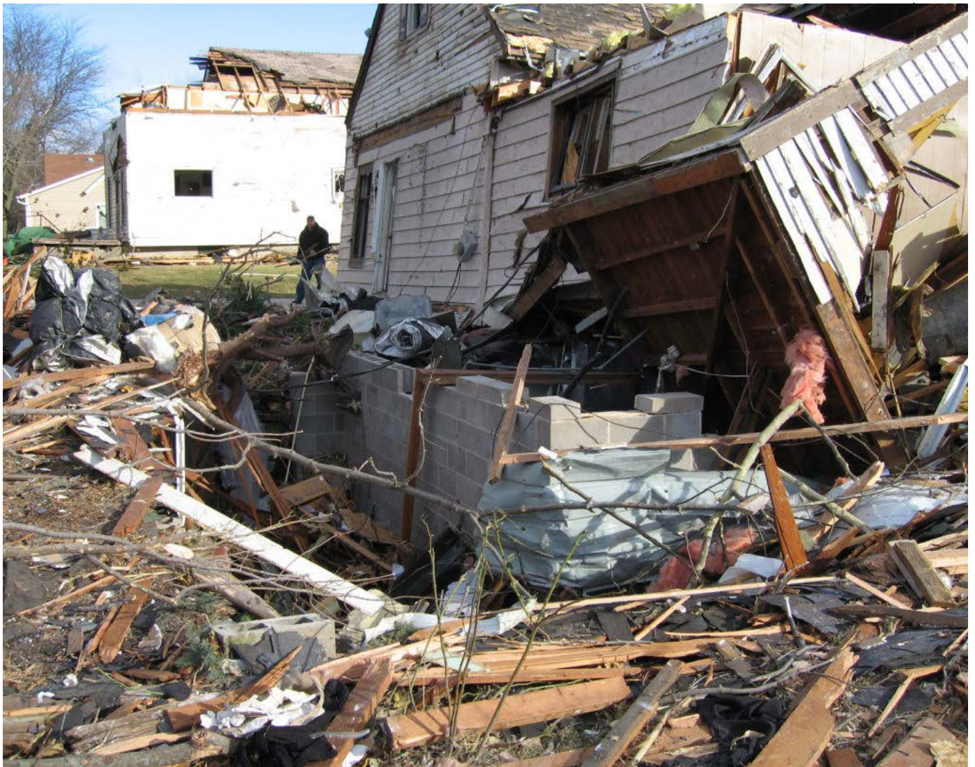
House slid off foundation in Woodward. F2 damage.
