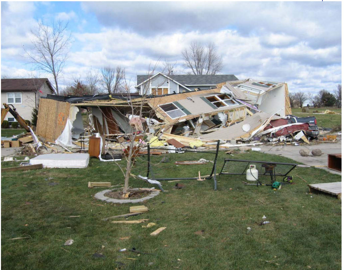
Double-wide home flipped on top in Woodward. F2 damage.
