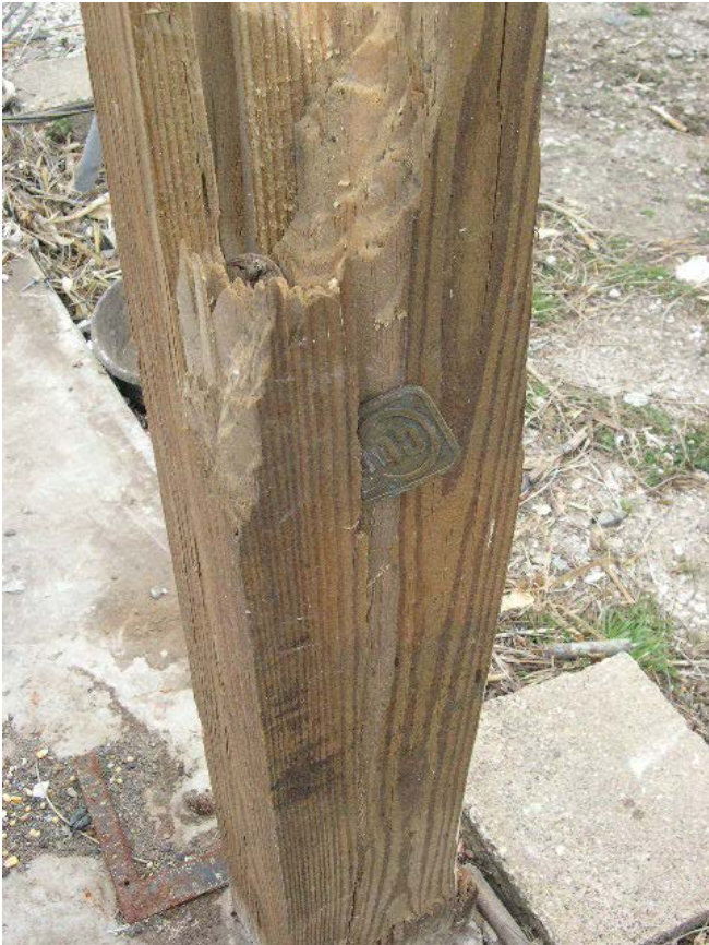
Belt buckle split post and became embedded in it near G Avenue in Webster county.
