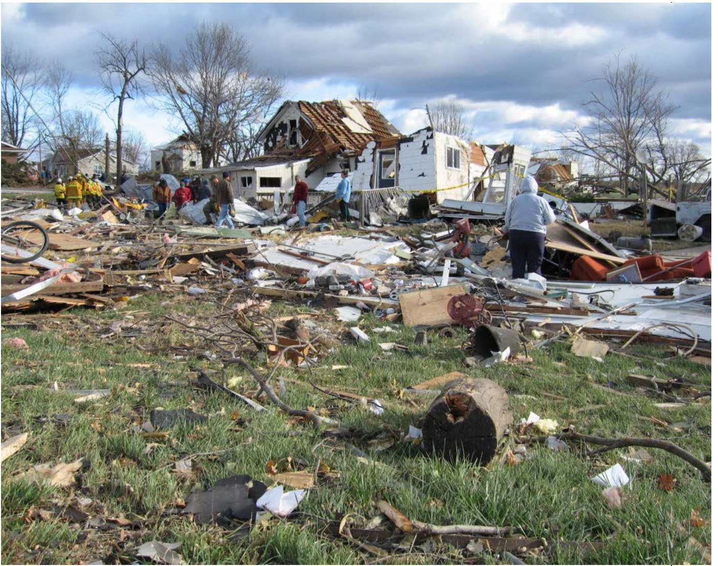
Flattened garages and damaged homes in south Woodward. F2 damage.
