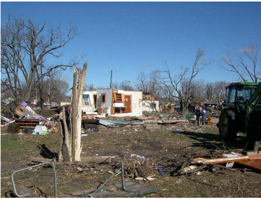
Homes heavily damaged throughout west central and northern sections of Stratford. F2 damage (preliminary).
