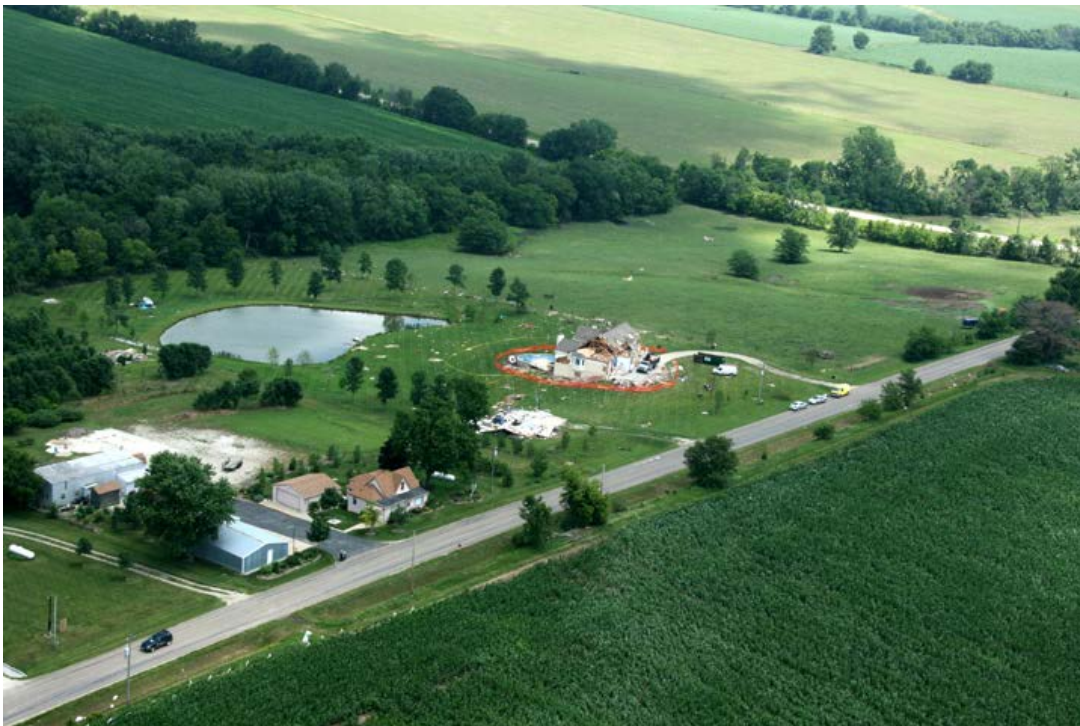
Aerial photo of home with EF2 damage southeast of Norwalk. The picture is looking northeast. Note the damage path in the corn approaching the home suggesting a northeast movement at this point. Courtesy of IowaHelicopter.com
