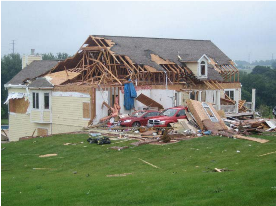
6) Home on the southeast side of Norwalk where the most intense tornadic damage occurred. The damage at this home was rated an EF-2 with windspeeds of 125 mph were estimated based on the damage.
