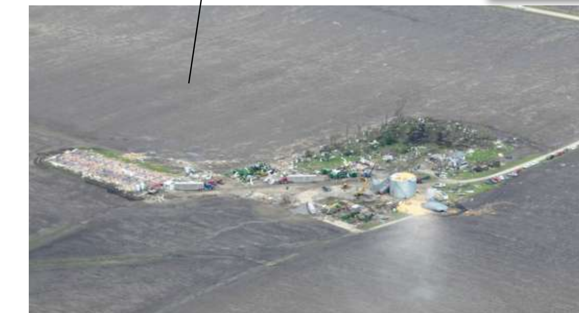
Damage on Lester Rd northwest of Dunkerton approached EF3 at several farm sites. Many hog confinement buildings were flattened. Here, hogs can still be seen in the building with some being loaded onto trucks. Civil Air Patrol photo.
