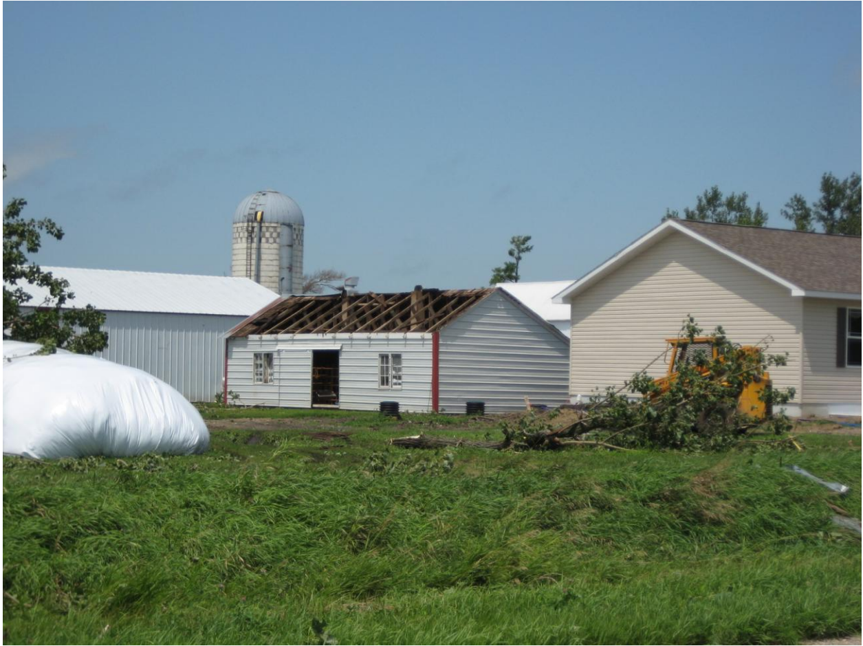
Figure 3. A building with roof damage near on the south end of Pocahontas.
