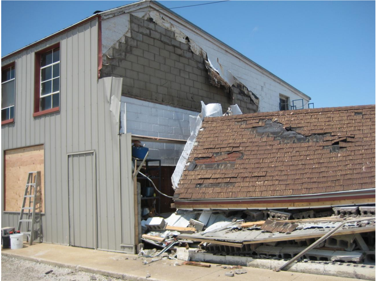
Figure 7. The cinder block wall of this building collapsed and the roof was torn off the side of the parent building in eastern Pocahontas.
