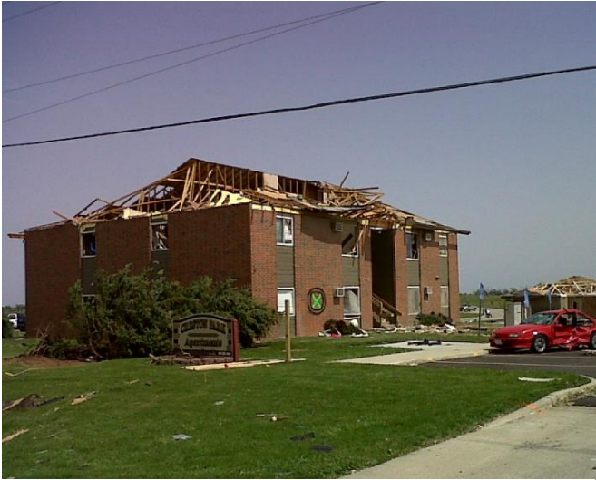
An apartment building sustained roof damage. Cars in the parking lot were dented and damaged.
