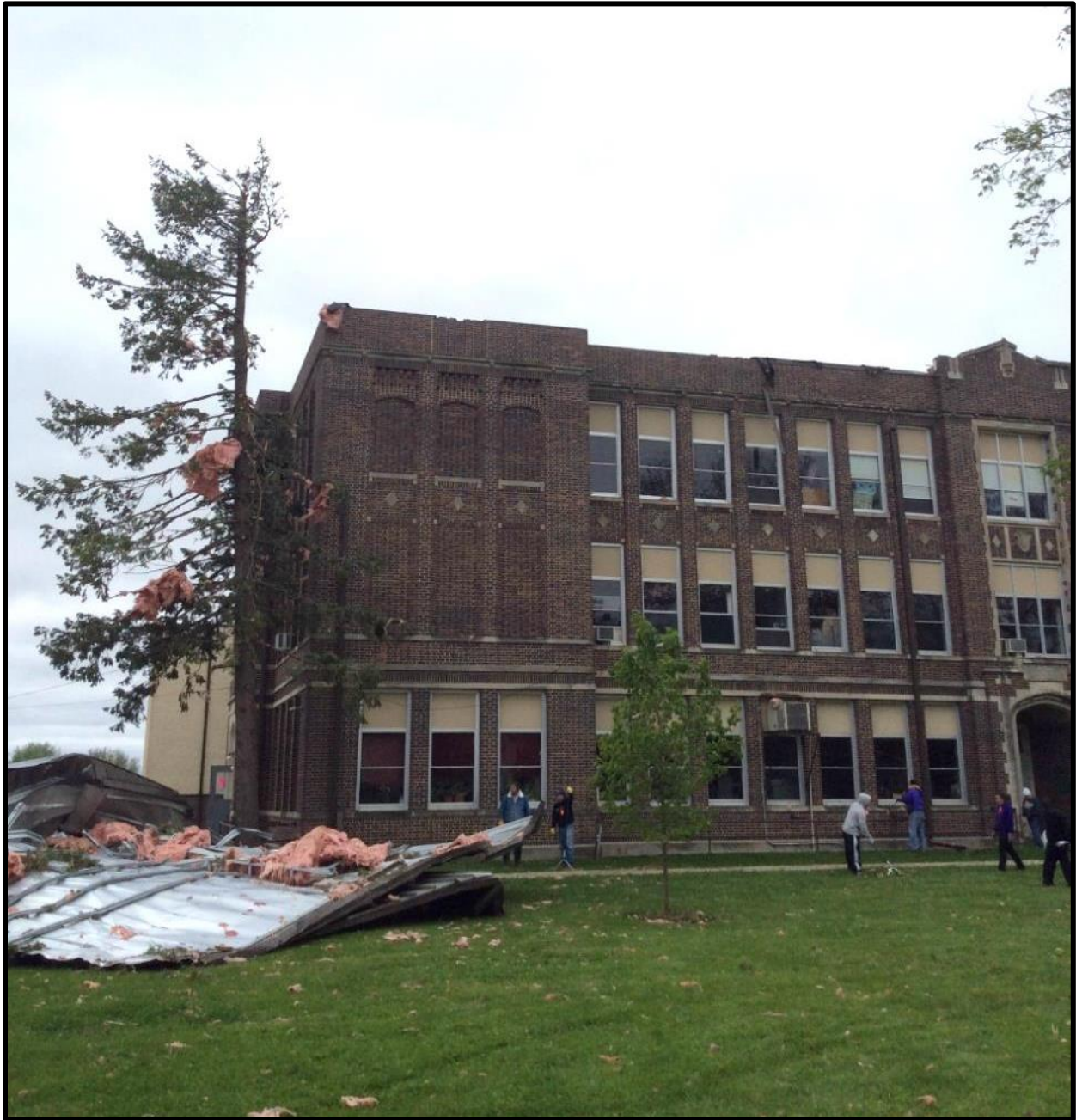
The roof was torn off the high school in Lake City. The tornado was rated a higher-end EF-1 with a maximum wind speed of 100 mph at this location
