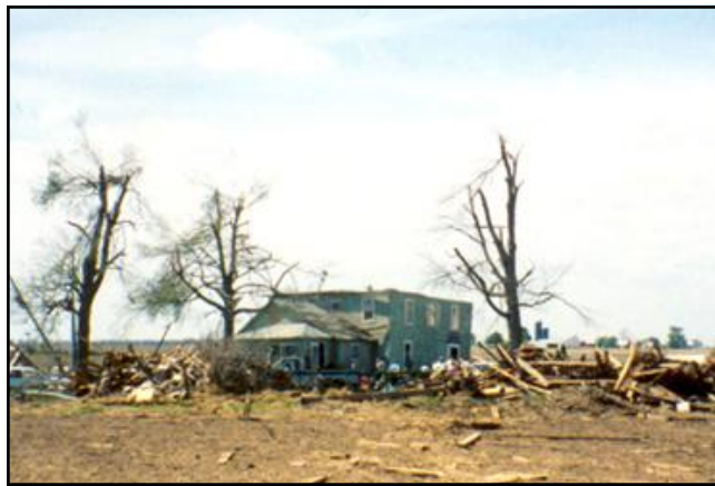
Damaged Illinois farmstead from the May 13, 1995 tornado.
