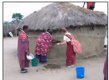
Adding a mud/cow dung mix to the siding of a boma (Source: Janine Vining)
