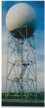
The Weather Surveillance Radar -1988 Doppler (WSR-88D) is the cornerstone of our warning operations. Being a Doppler radar, it allows us to "see" wind motion in storms which can signal the early stages of tornadoes, damaging winds and large hail. Use of the WSR-88D has significantly improved the warnings issued by the NWS. Although its name implies it was built in 1988, its software and hardware are continuously upgraded to keep pace with current technology and science.
