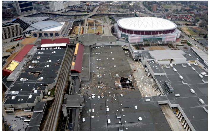
Georgia World Congress Center damage caused by the March 14 tornado. The SEC championship basketball game was underway in the Georgia dome (top) at the time. A tornado warning was issued 8 minutes prior to the tornado's first damage. (Photo courtesy Atlanta-Fulton EMA.)
