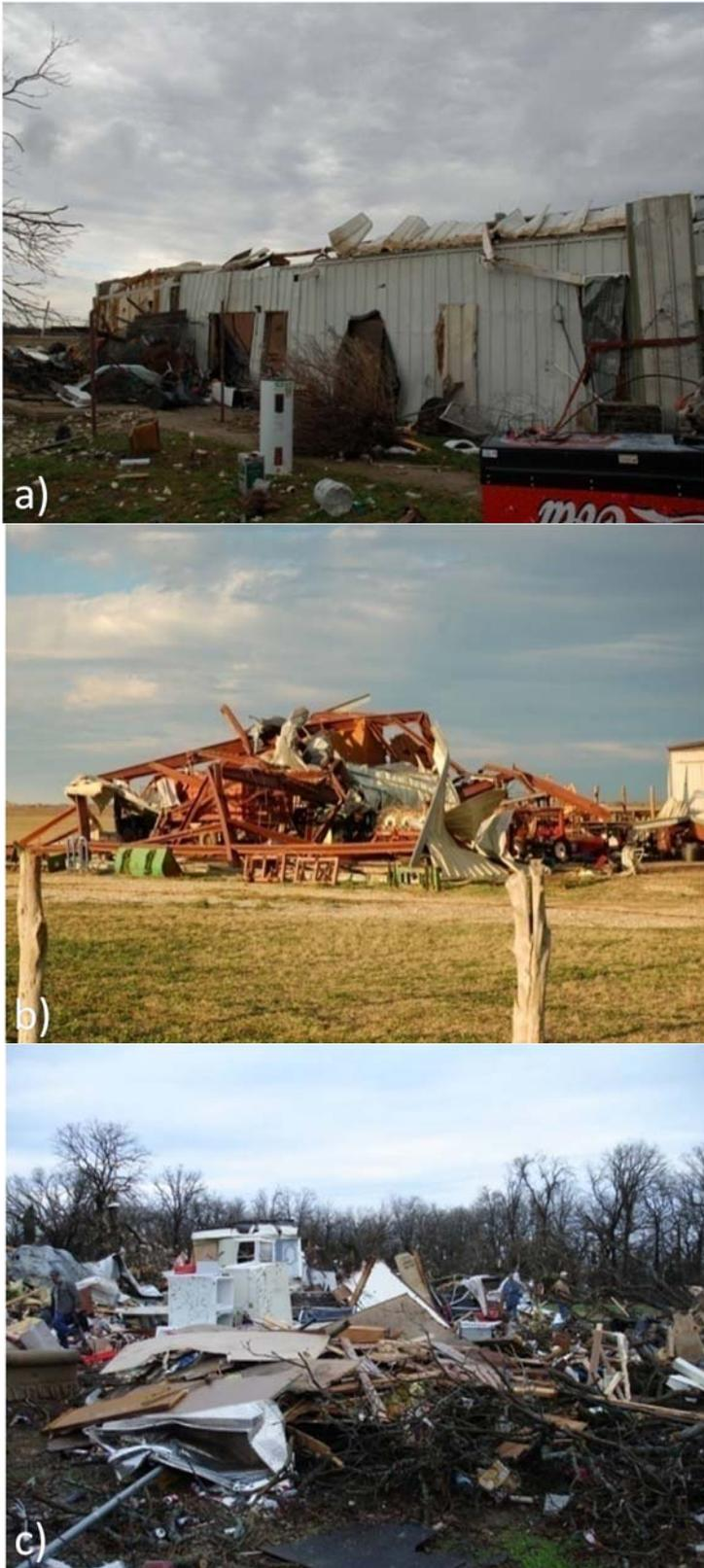
**Fig 3.** Photographs of damage caused by tornadoes on 29 December 2006. (a) Significant damage to a retirement home for veterans located outside of Groesbeck in Limestone County; (b) Damage to a metal framed barn east of Clifton in Bosque County; (c) Remains of a mobile home destroyed by a tornado northeast of Rio Vista in Johnson County (Photo courtesy Gerald Mohr, Johnson County Emergency Management Coordinator).
