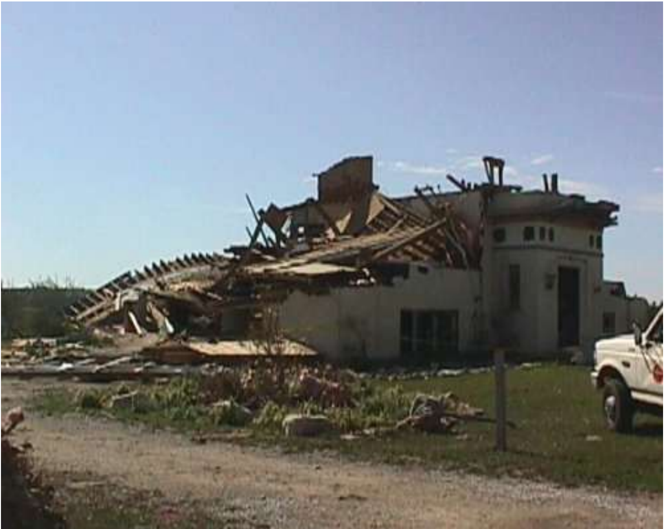
This building (left picture) was on the south side of the tornado as it passed over Hwy 42 (Photograph by Jill Last, NWS Green Bay). There used to be a farm house and barn here (picture on right).
