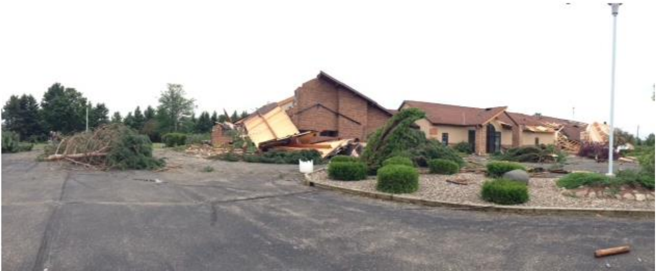
Figure 1: Church (southeast New London) damaged by a tornado. Peak winds were estimated at 115 to 120 mph.
