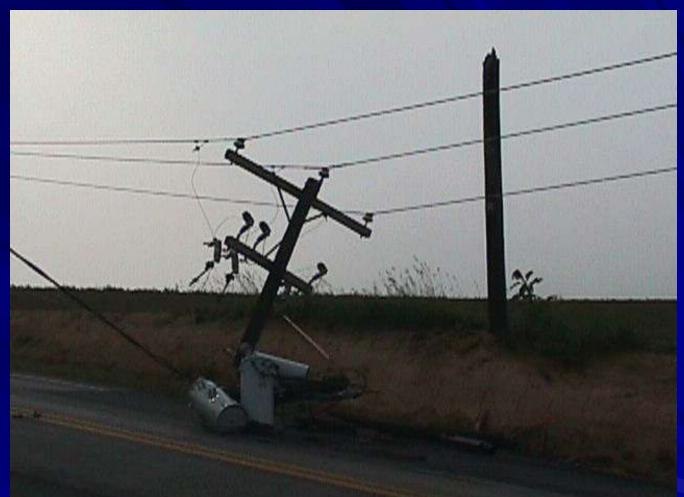
Either trees falling on wires or force of wind against wires in open country can cause poles to snap. Very difficult to estimate wind speeds needed to do the latter.
