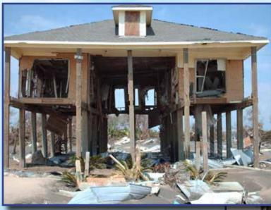
Storm surge flood damage near Caplen, TX. Note house destroyed from flowing water from bottom up. Photo credit: NOAA/NWS.
