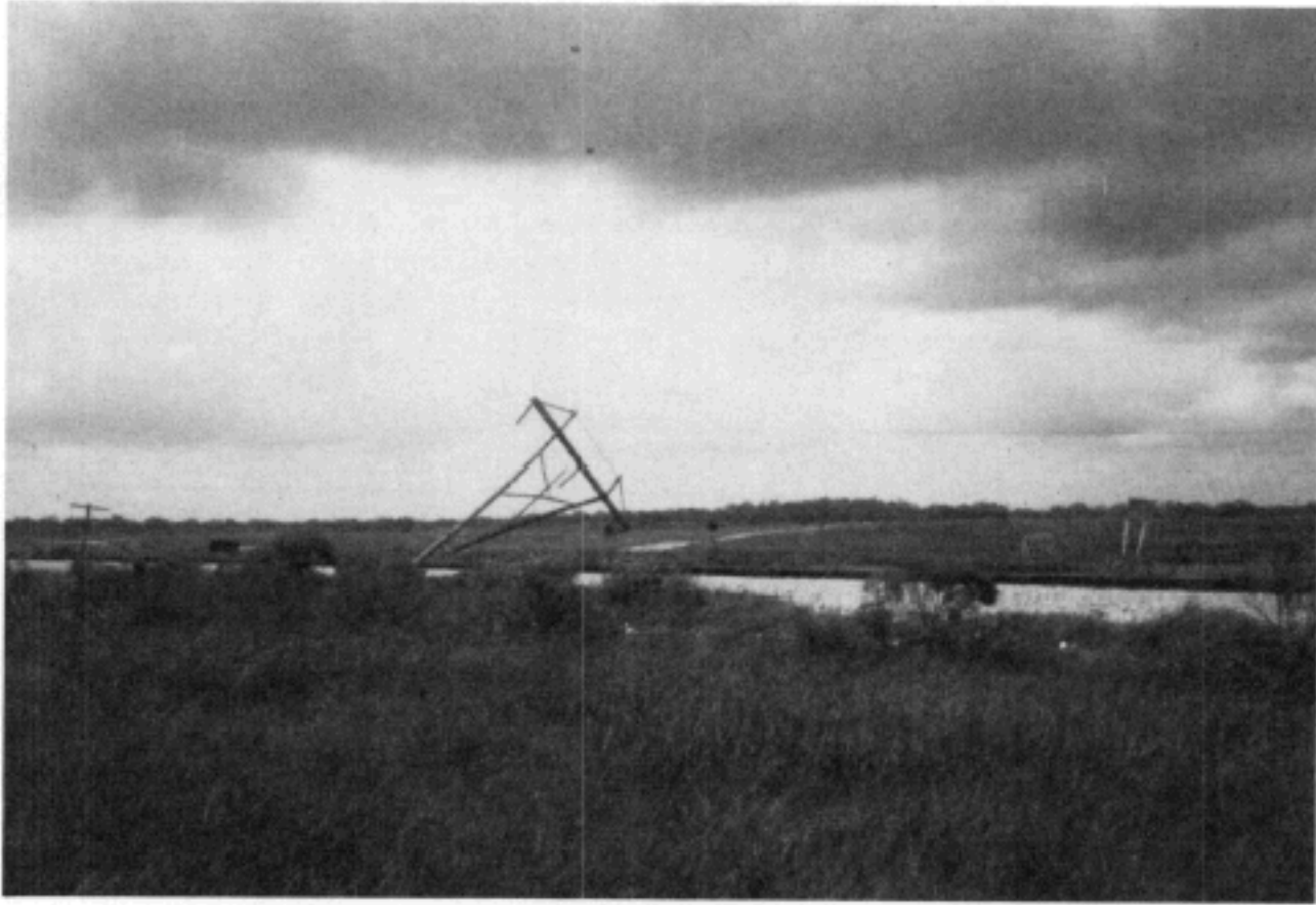
FIGURE 5.6 Failure of primary power pole near Highway 146 south of Bay City.
