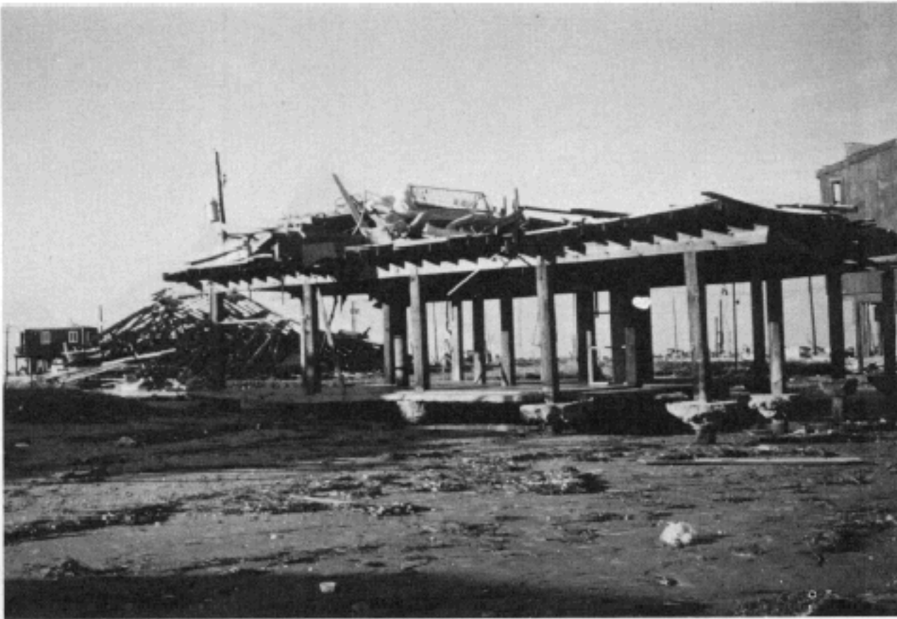
FIGURE 4.43 Example of a superstructure blown away by the wind. A mound of lumber, furniture, and appliances is in the backyard of the house.
