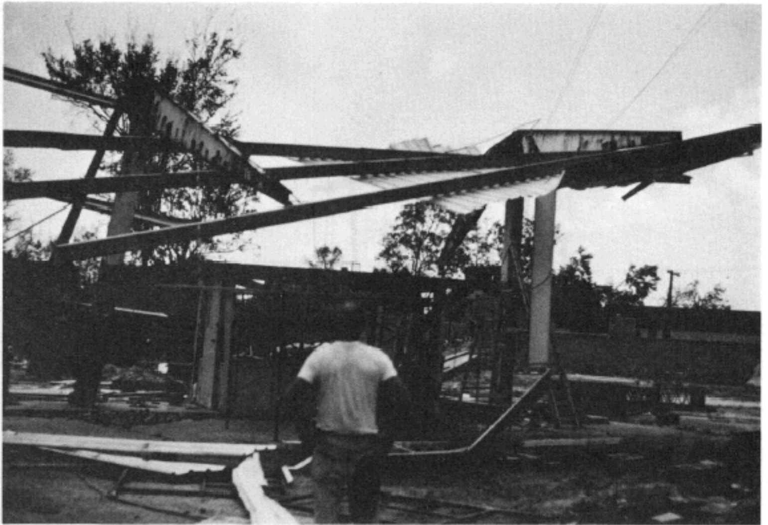
FIGURE 4.16 Failure of sheet metal roof at a gas station.
