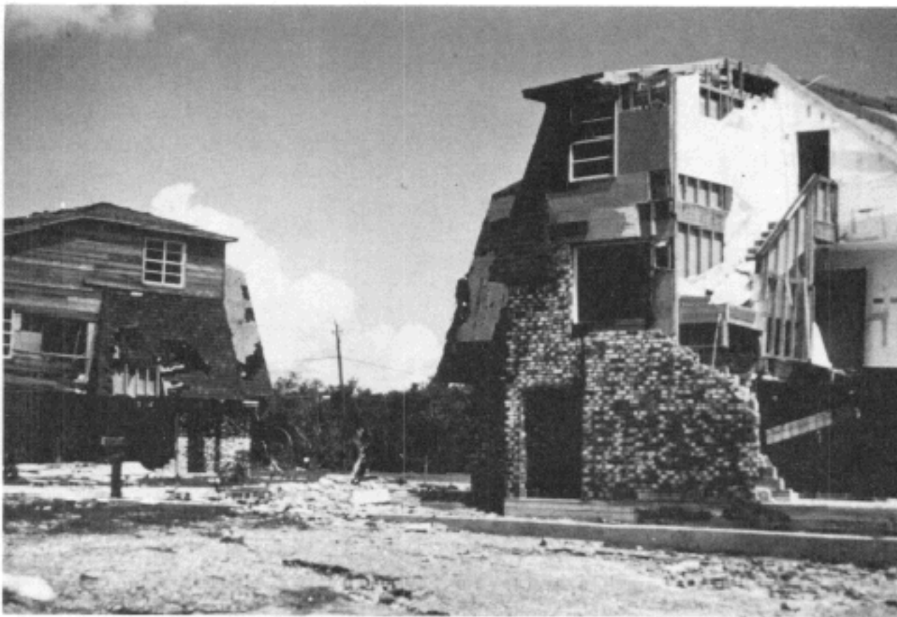
FIGURE 4.59 Failure of the roof and brick veneer wall of a condominium.
