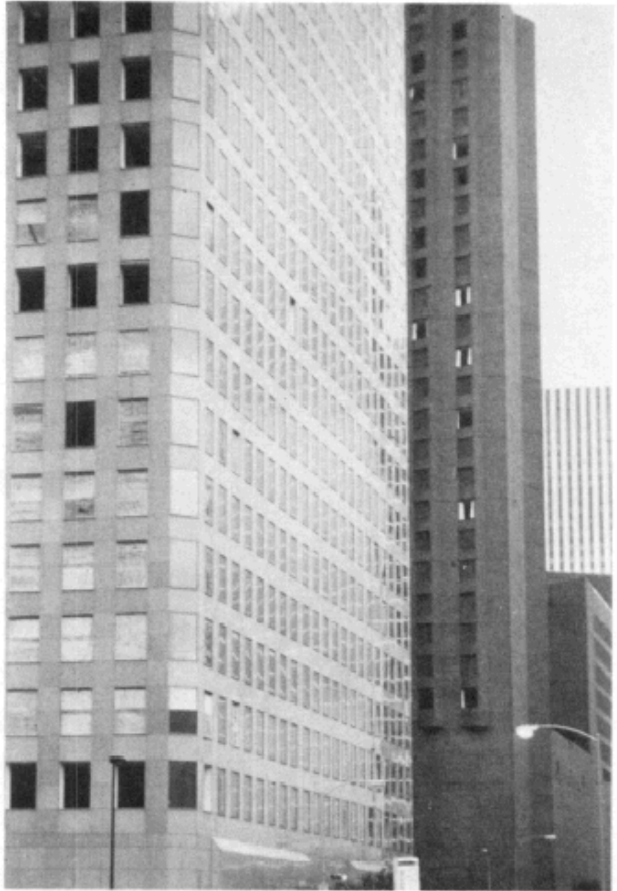
FIGURE 4.7 Window damage to the Hyatt Regency Hotel (the building in the background).
