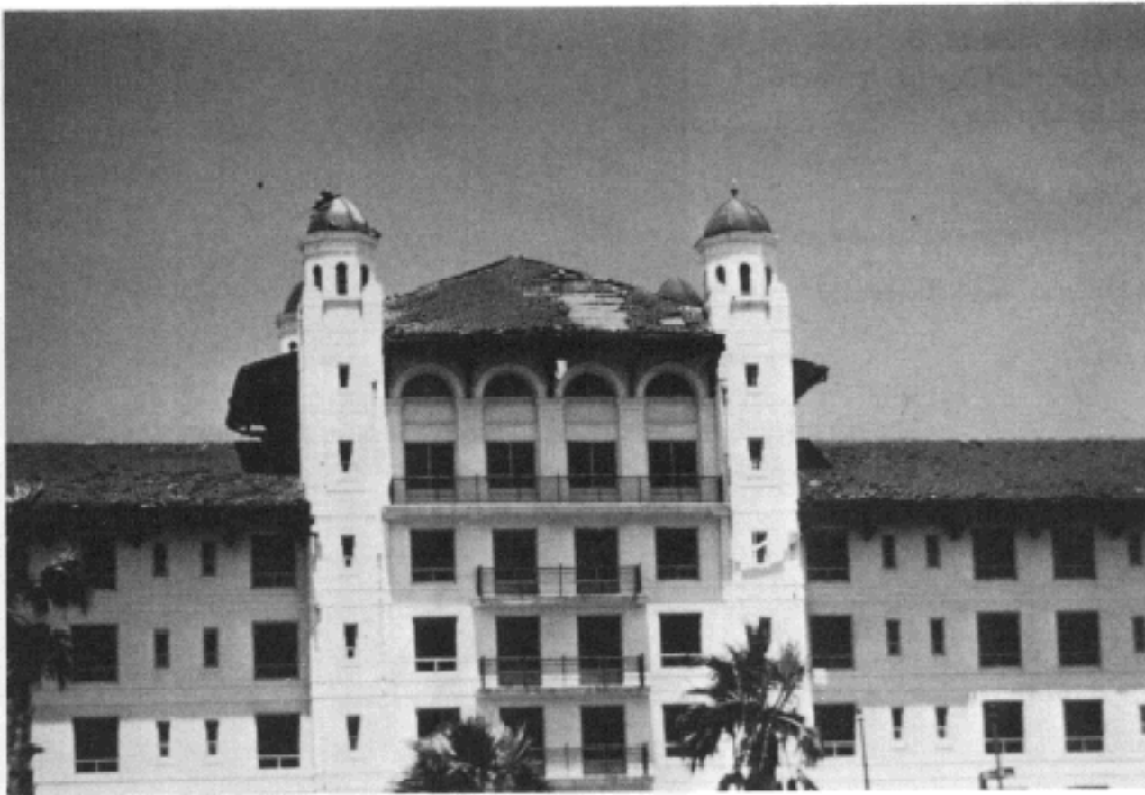
FIGURE 4.22 Damage to tiled roof of the Hotel Galvez.
