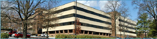
NSSTC Building (location of NWS Huntsville)
