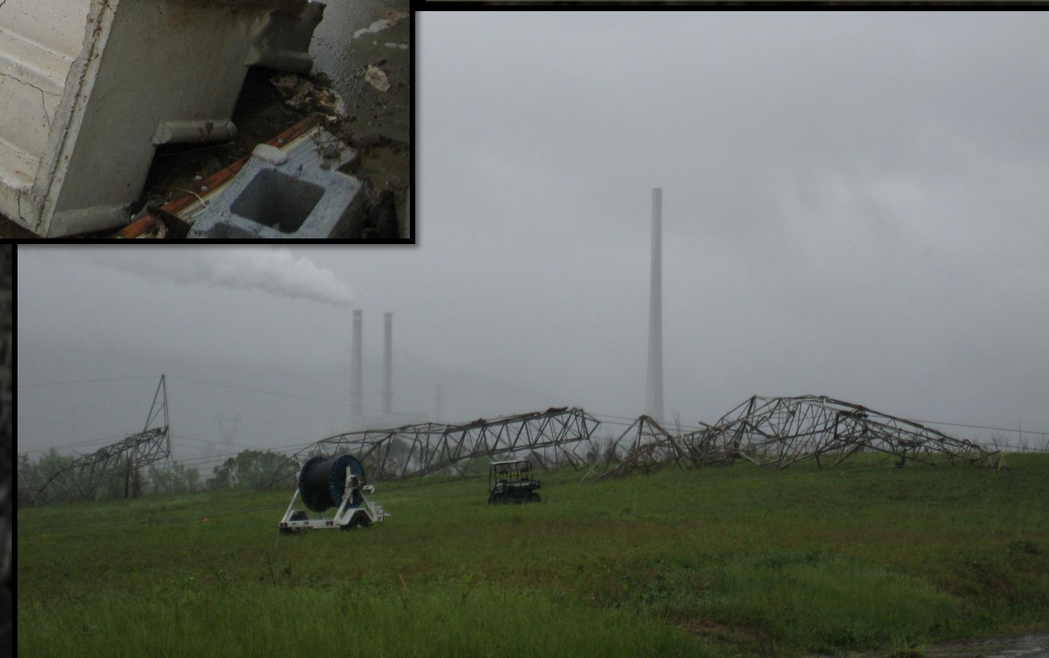
Damage photos (right) show a demolished house down to its foundation, as well as high-tension electrical truss towers crumpled. To the left, a map of the tornado track is shown.
