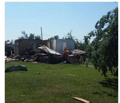
Damage in Eureka, from storm survey
