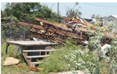
Damage in Eureka, from storm survey
