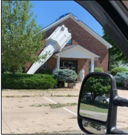
Figure 6. Wind damage in Oswego. Photo courtesy of Labette County Emergency Management.
