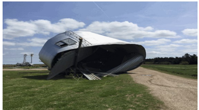
Figure 3: EF1 damage southeast of Ellinwood.
