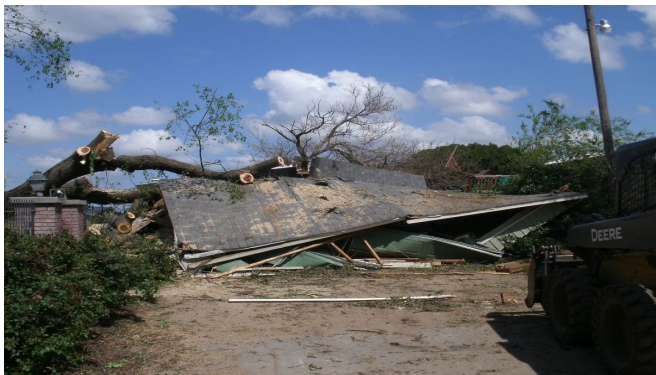
Figure 2: EF1 damage southwest of Nickerson.
