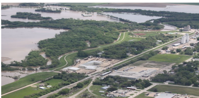
Figure 5: A levee system around the town of Halstead holds back the swollen Little Arkansas River in May.
