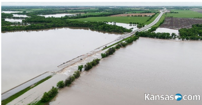
Figure 4: A portion of the Kansas Turnpike south of Mulvane closed in early to mid-May due to the swollen Slate Creek. A Turnpike closure of this magnitude and extent due to flooding hadn't occurred in over 30 years.
