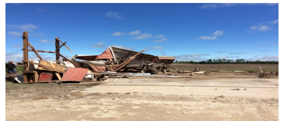
Figure 3: Tornado damage to a farmstead northwest of Waldo.
