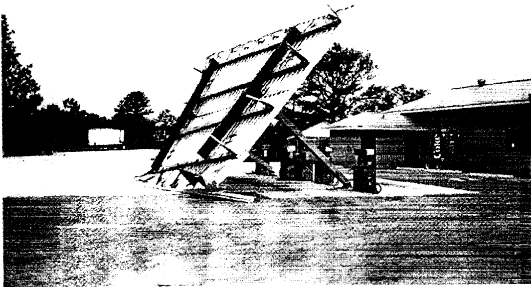
Figure 8. Gasoline Pump Canopy, US 421 Northwest of Wilmington.
