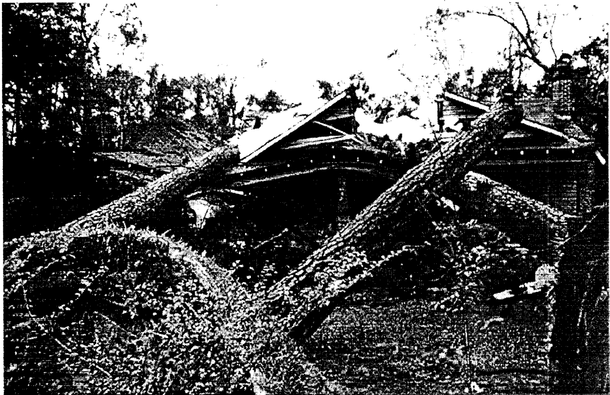
Figure 9. House Damage by Fallen Trees Along US 17 Northeast of Wilmington.
