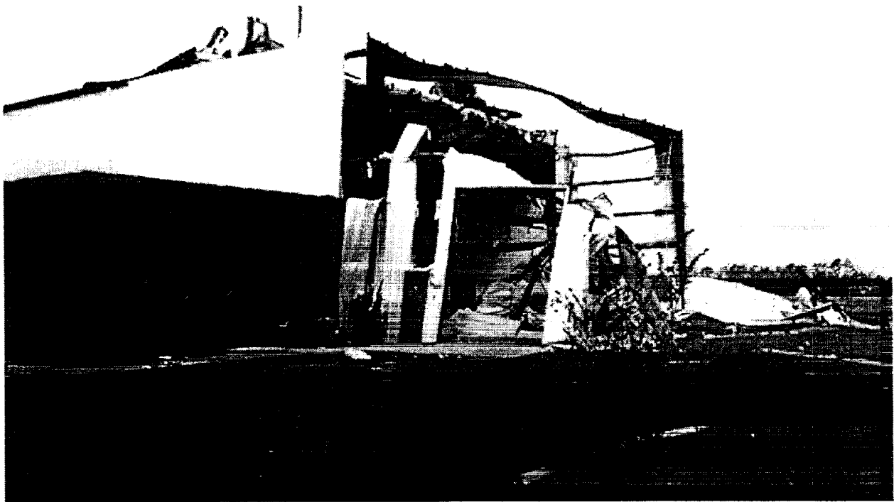
Figure 6. Aircraft Hangar, Wilmington International Airport (view to northwest).
