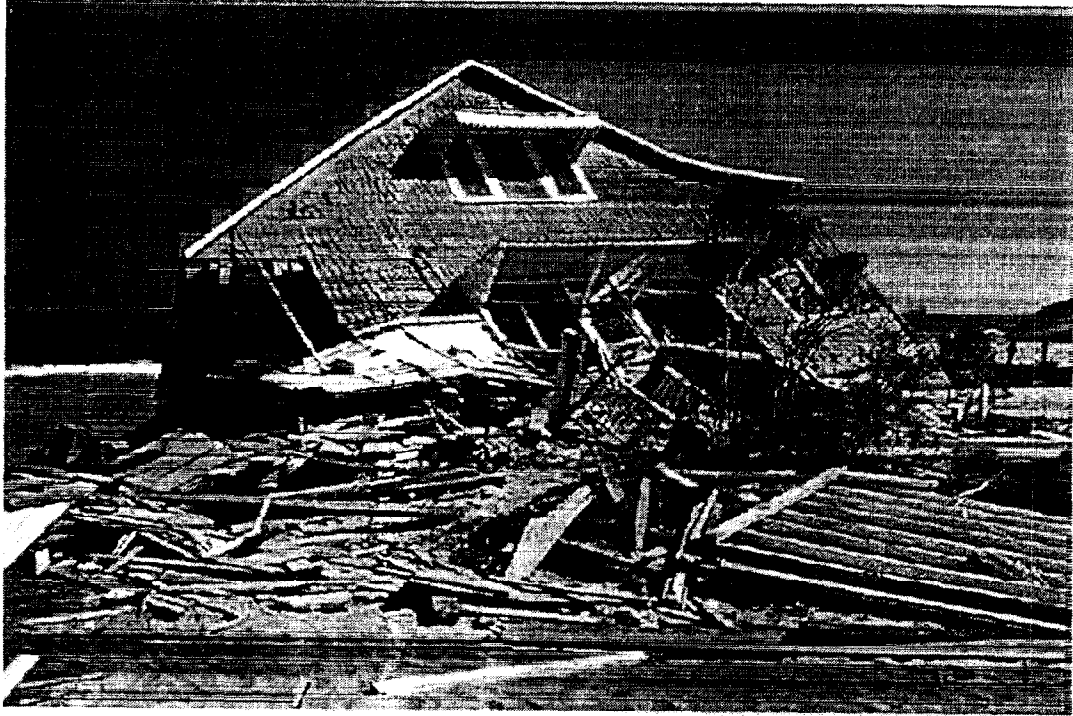
Figure 3. Surge and Wave Damage, North Carolina Coastal Area (Source: FEMA).
