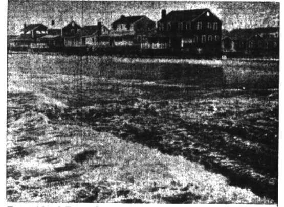
The crooked wood piling seawall constructed in front of these cottages at Money Island proved its worth during Helene. At no time during the storm did breakers go over the wall.
