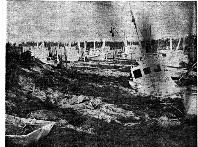
Boats moored along the thoroughfare between Cedar Island and another land, are in deep water. Dead marsh grass was floated across the road and is one to three feet thick on top of the water. The road was blocked for a time by the marsh grass, at some places 4 feet deep on the hard surface.
