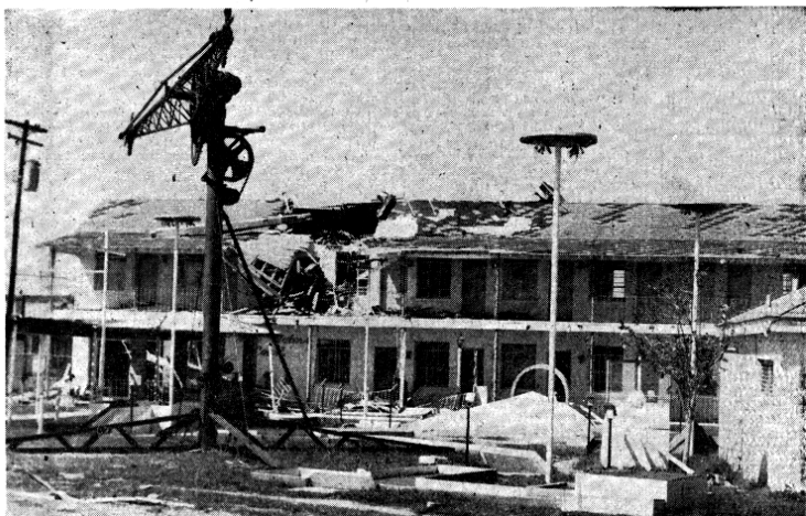
MAMMOTH CLEANUP — Areas hit by Helene Sunday faced the backbreaking job of cleaning up. Above, at Carolina Beach, one of the spots hardest hit, a roof was ripped from a building and thrown more than a hundred yards through the roof of this motel. Winds did more damage than water.
