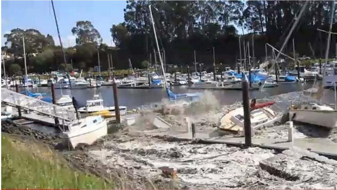
*Figure 7 Photo showing one of several single, amplified waves that entered into the back half of Santa Cruz Harbor, causing damage to a number of docks and boats (from Wilson and others, 2012a).*
