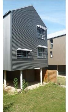
Figure 1 : Example of two-storey house built on stilts. Saint-Pierre-des-Corps, France (CEPRI)
